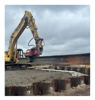
The main construction of this feature is now complete and the sheet piles which formed the working area around it have now been removed.
